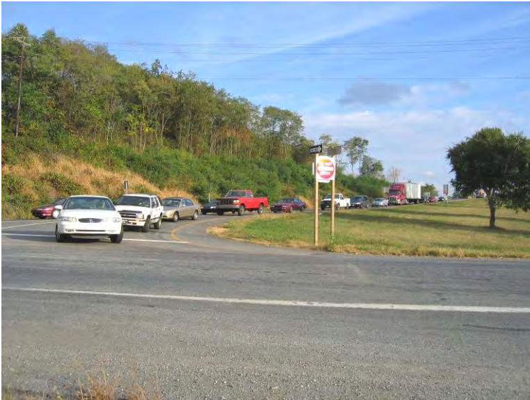
Queues on Ramp B (Route 283 westbound off-ramp) extend approximately 700 feet during the weekday P.M. peak hour under existing conditions.
