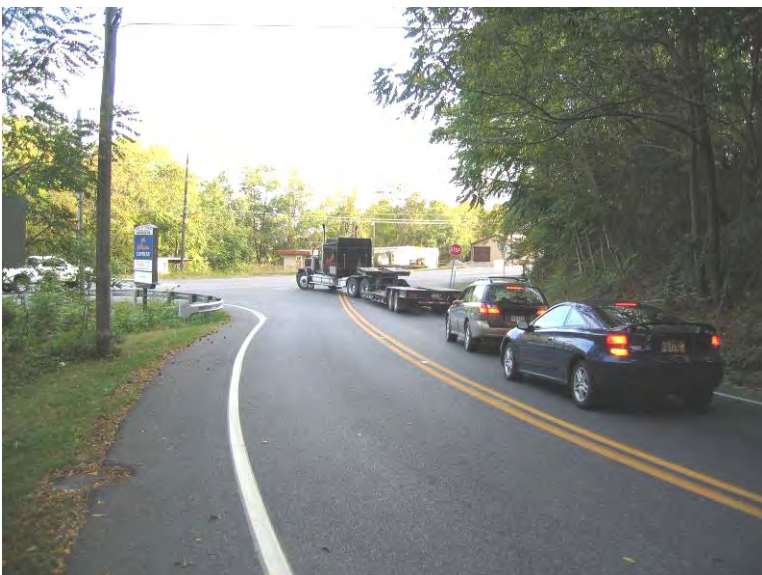
Excessive delay occurs on stop-controlled approaches of intersecting roadways with Cloverleaf Road.
