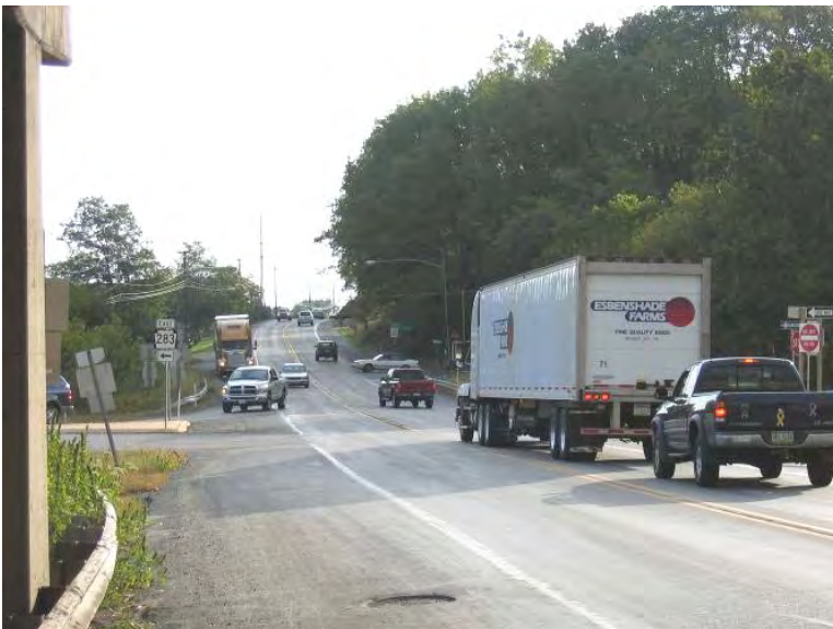
The lack of left turning lanes on Cloverleaf Road at the intersections with the Route 283 ramps causes delay to through vehicles.
